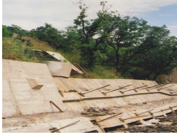
Figure 2. Photograph of anchor against landslide construction, installed in Crimea
